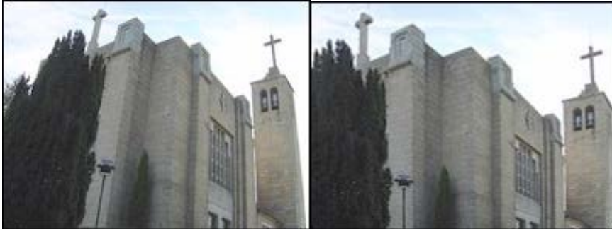
Straightening of the lines of leaks.
